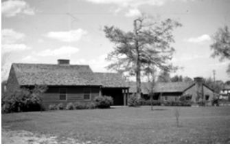
House and Shop at Great Circle ca 1937
